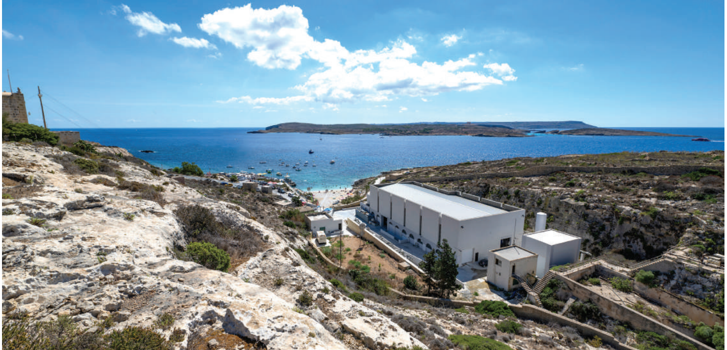
The Hondoq RO Plant in Gozo has been honoured with the esteemed Energy Globe Award, a testament to its pioneering methods in seawater desalination.
